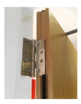
During the operational life time of a fire resisting door, it is possible that the intumescent seals around the perimeter of the door will become damaged or removed by wear and tear, impact or intentional vandalism.
